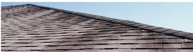
This 8-year-old roof in Florida is an example of a roof where algae-resistant copper granules are not present in the hip and ridge shingles.
