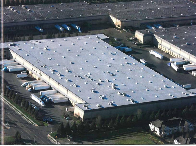
longer." The wood fiber cover boards were mechanically fastened with screws and plates using 12 fasteners in the field, 15 fasteners on the perimeters, and 24 fasteners in the corners.
